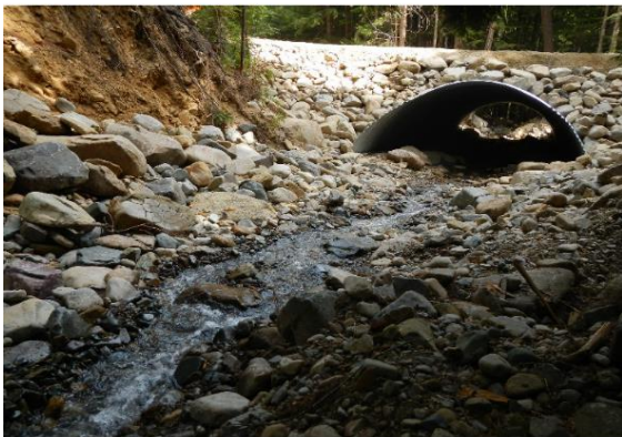
Completed bottomless arch— looking downstream
